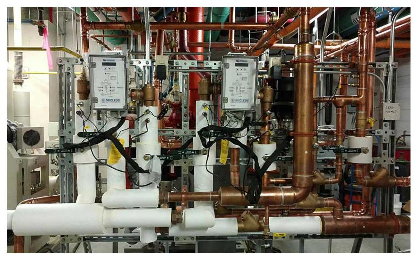
Manufacturers are supplying today's better performing digital mixing valves stacked with features and enhancements that carry the capabilities of remote temperature adjustment, high temperature sanitization, building management system integration, multiple temperature and pressure measurement points, flow measurement, self-cleaning, self-monitoring and self-balancing. Photo courtesy of Leonard Valve.
